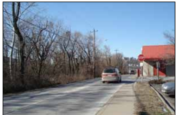
Riviera Drive at Site of Proposed Off-Ramp Intersection
